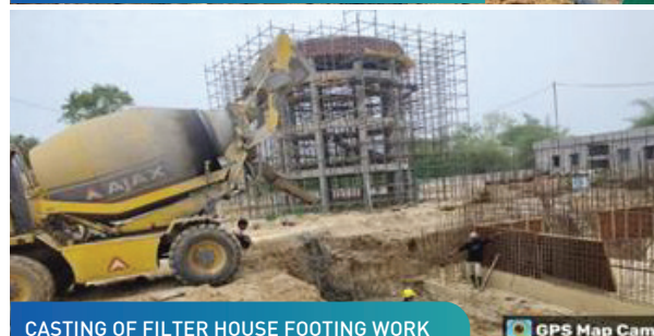
CASTING OF FILTER HOUSE FOOTING WORK
