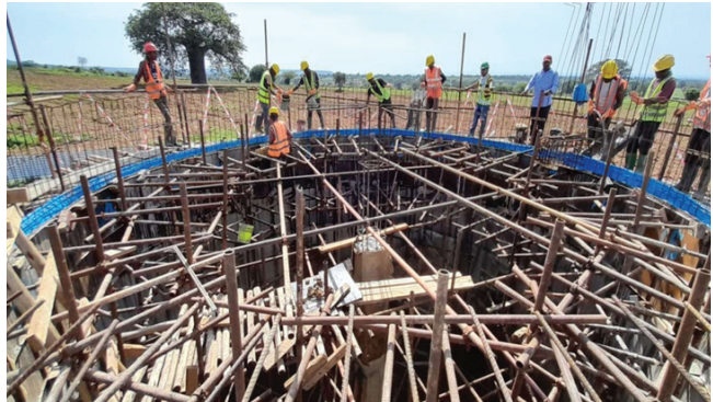
4th Lift wall concreting at Mgela GSR – 250cum
