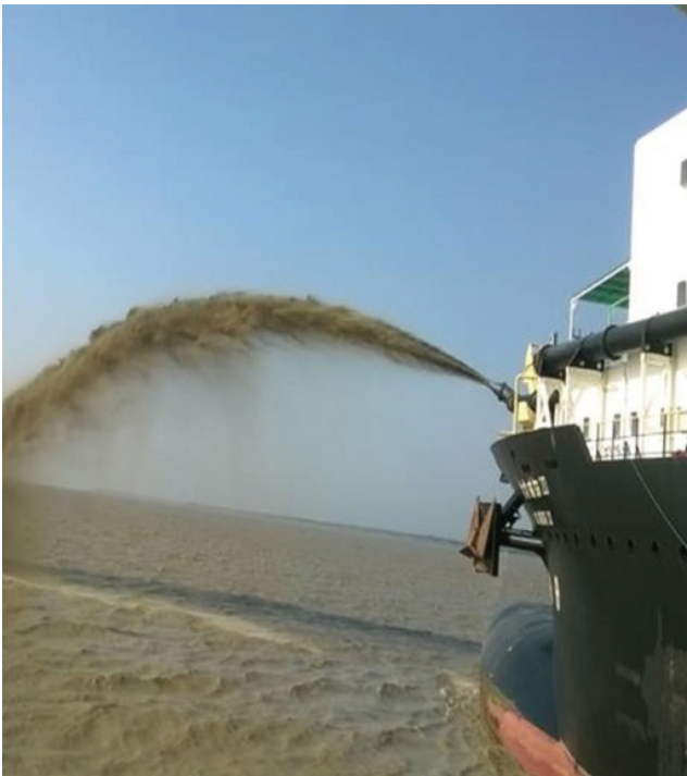
Dredging by Rain Bowing Method
