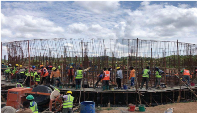
1st Lift wall concreting at Buchama GSR – 1150cum
