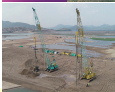
Vibro Compaction at Dam Footprint of Gap II (ECRF Dam)
