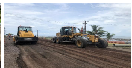
Construction of Subgrade improvement layer in progress
