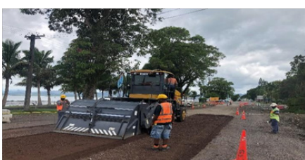
Pre-hoeing of Existing AC surface along QED
