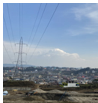
Under-construction 132/11kV Phutung Substation in Kathmandu Valley
