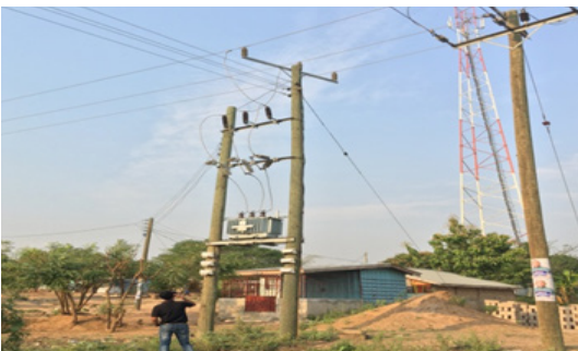
Existing Tapping & DTR Arrangement
