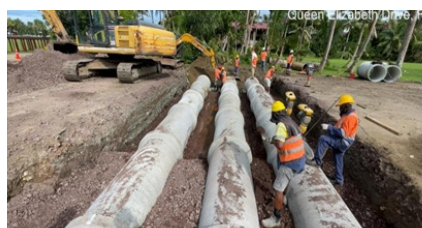
Inspection of Culvert installation works along Queen Elizabeth Drive Road
