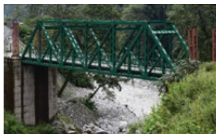
Completed Bridge Work
