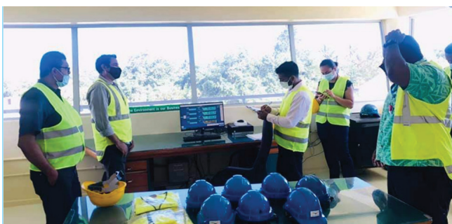
Kinoya WWTP Plant visit with Ministry of Economy officials and briefing by Country Manager about the plant works progress at SCADA Room
