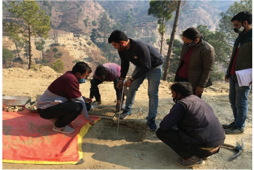
Checking of Thickness of GSB Layer
