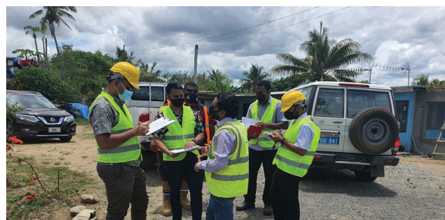
WAPCOS Engineer site visit with Ministry of Economy officials at Black Sewer Rising Main Project Nadi
