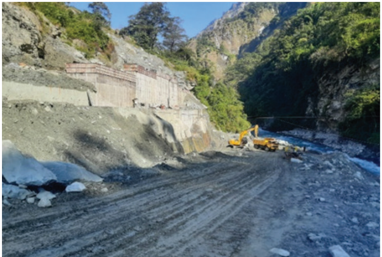
Concreting Works in Barrage Protection Wall
