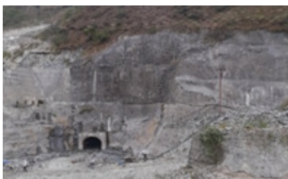
Excavation Work in Powerhouse
