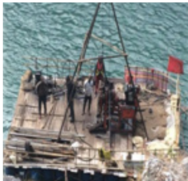
Core Drilling at Regulating Dam Axis
