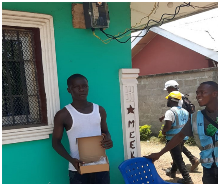
Energy Meter Installation
