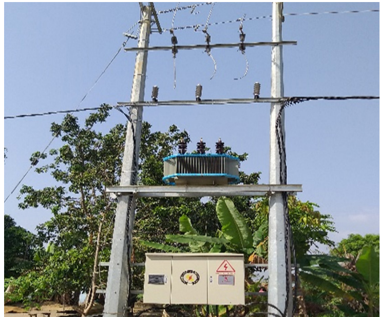
Distribution Transformer Installation
