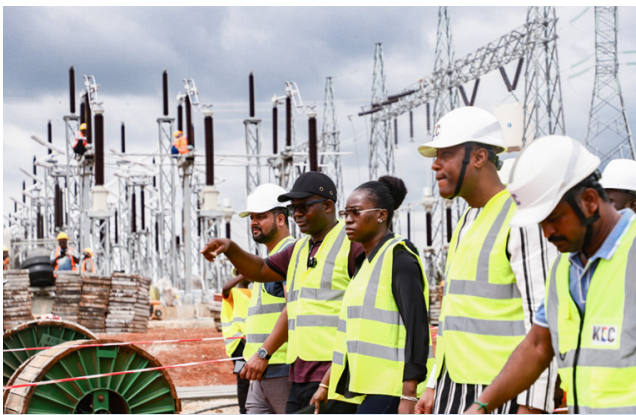
Distribution Transformer Installation
