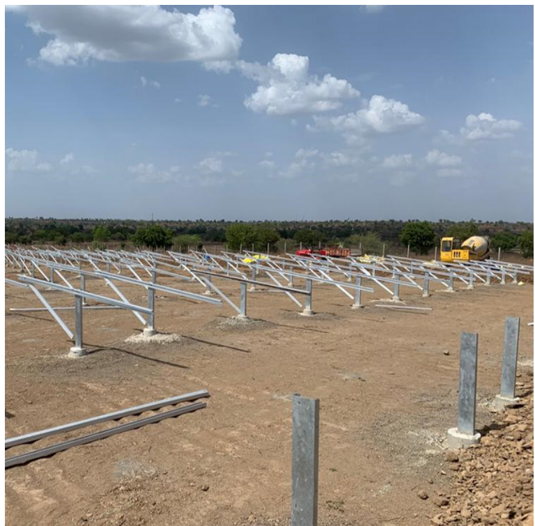
Module Mounting Structure (MMS) installation
