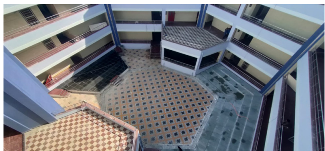
Inside View of Hostel Building
