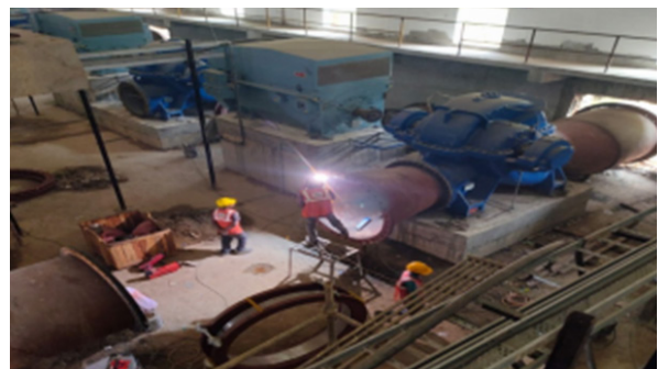
Erection of Reducer at Pump Discharge Portion in Progress at TURUNGA PS-01, GMLI Project.
