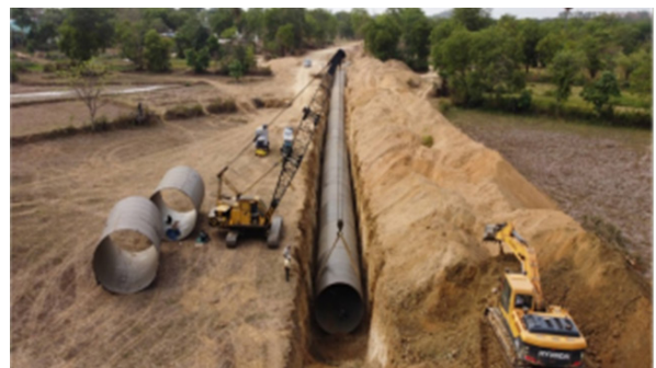
Excavation , Laying and Jointing work in progress for MS Line (2.6 M Dia) at Distribution area , GMLI Project.
