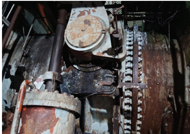
Deteriorated condition (MIV) due to water leakage and ageing effect
