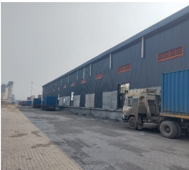
Completed outside PEB cladding works with skylight and Louvers
