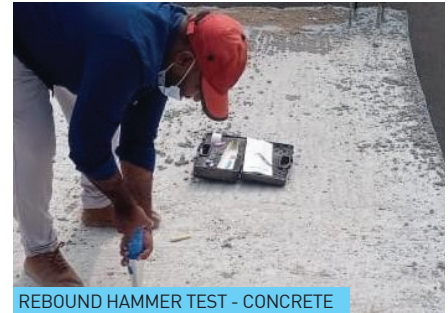
REBOUND HAMMER TEST - CONCRETE
