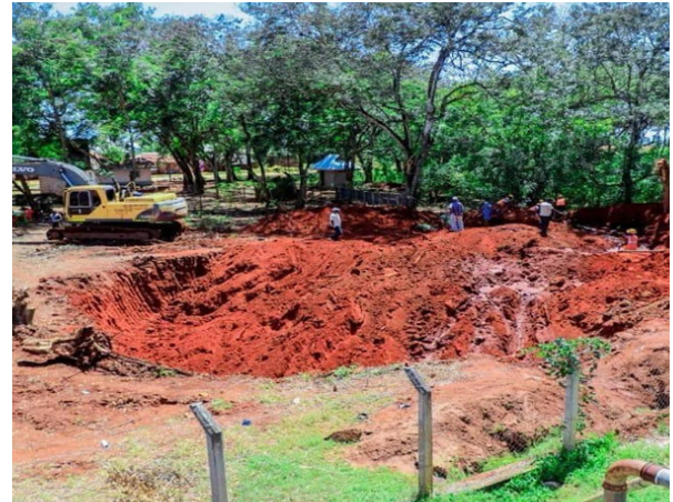
EXCAVATION IN BOZA ESR 500CUM
