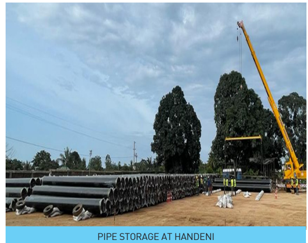
PIPE STORAGE AT HANDENI
