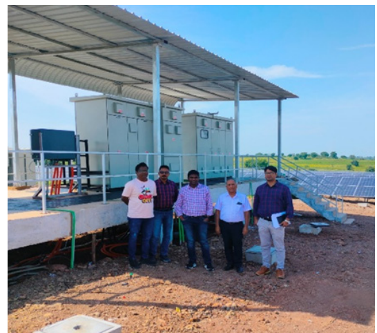
PMA and Client PFC Teams Joint Site Inspection
