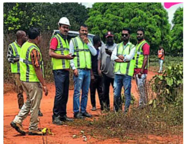
DURING CLEARANCE OF ROW OF CWTM
