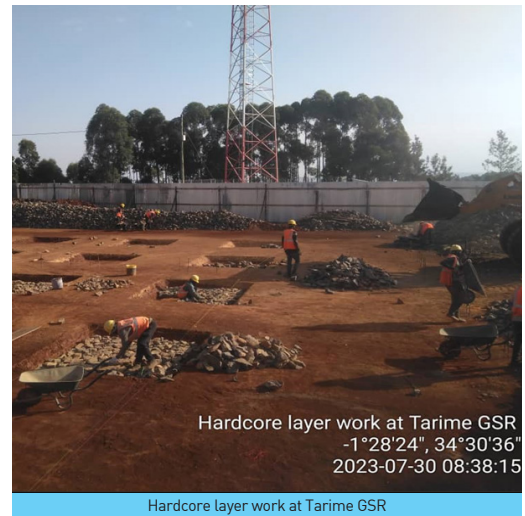
Hardcore layer work at Tarime GSR
