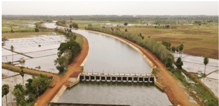
PMC for ERM of Grand Anicut Canal Project - Construction of New Regulator @ LS 29900 M
