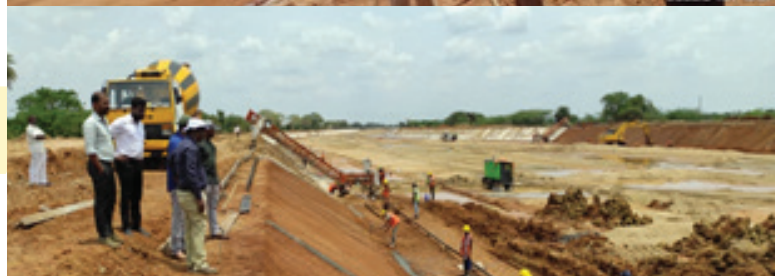
PMC for ERM of Grand Anicut Canal Project – Lining of GA Main canal
