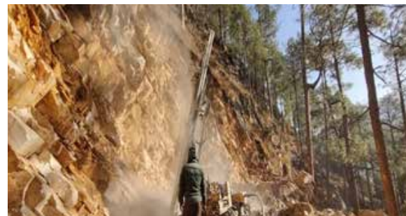
Hill side cutting work in progress
