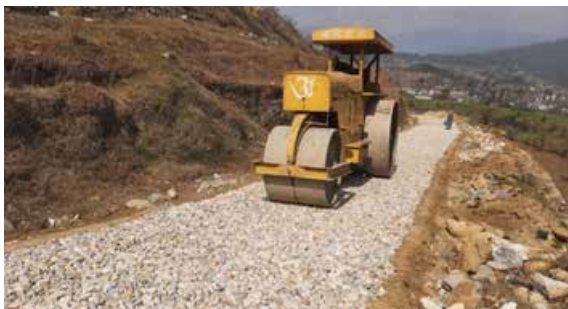
Laying and Compacting of GSB Layer
