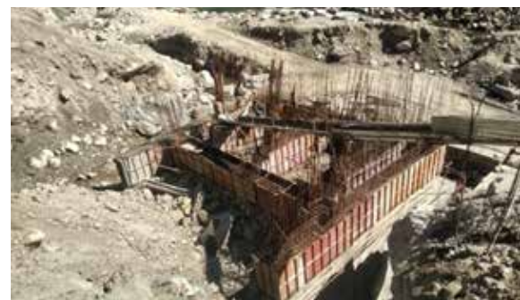
Construction of RCC Bridge Abutment in progress
