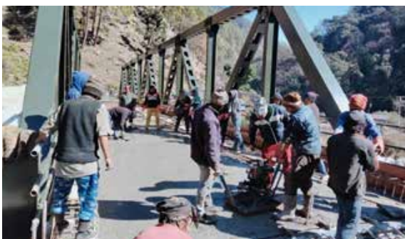
Laying of RCC Slab in Bridge
