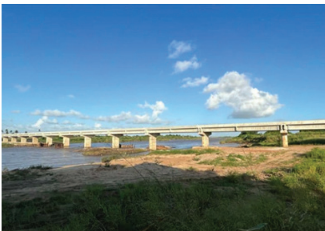
Buzi River major bridge of 690 m length completed
