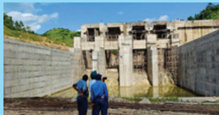
Spillway Blocks 3-4 (Radial Gates Erection underway)
