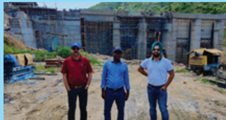
Dam Blocks 1-4 (completed till top)
