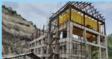
POWERHOUSE: EOT Commissioning and Truss Erection underway
