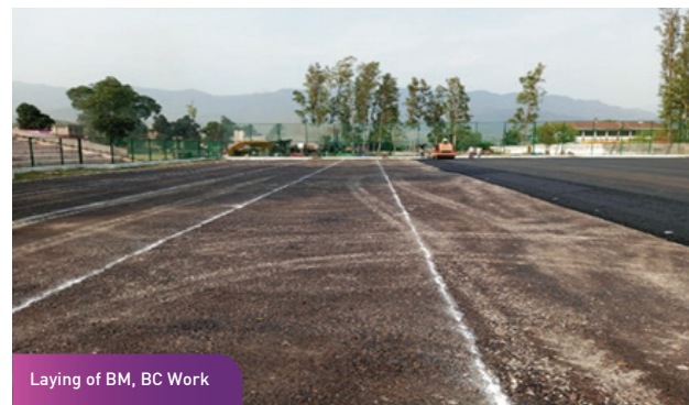
GSB Laying and Compaction Work
