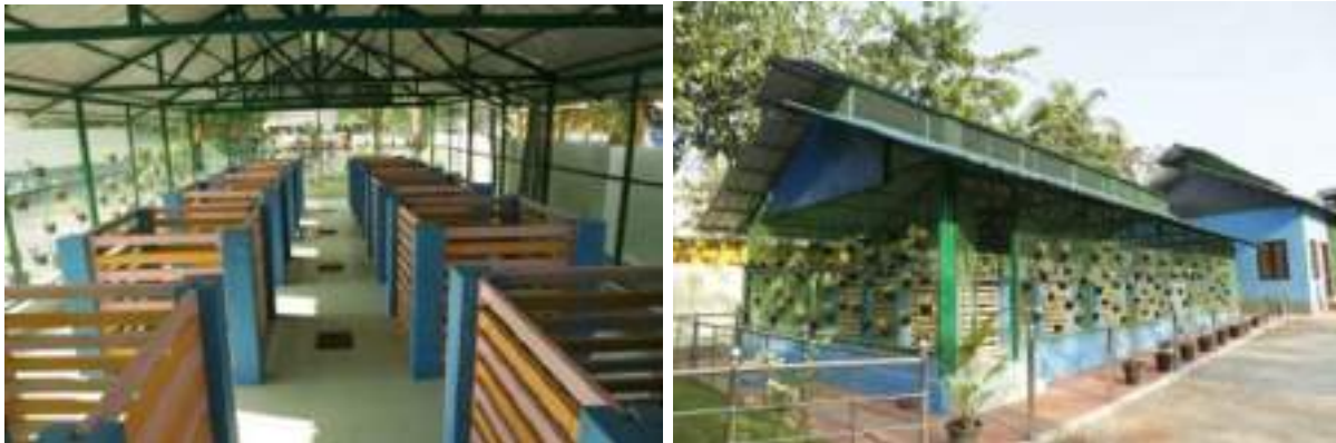
Figure 8-17 Thumboormuzhi aerobic compost unit
