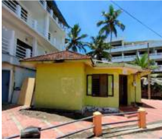
Figure 4-9 Existing toilet to the southern end of light house beach
