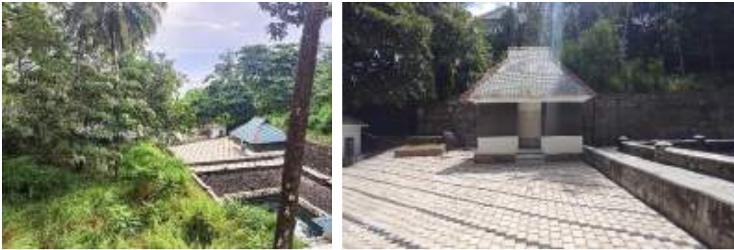
Figure 4-6 View of Silent Valley Sub Bath Park (left); Toilet block in Sun Bath Park (Right)
